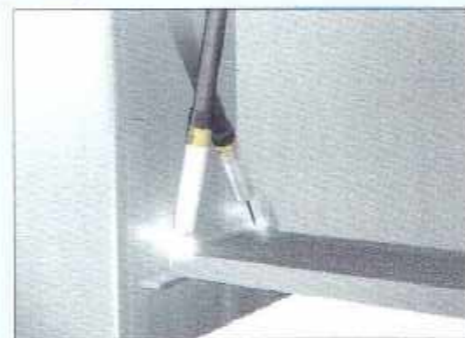
▲ for Fillet welding in a tight space
